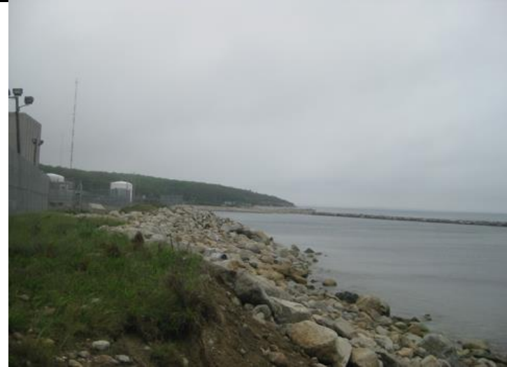
View looking north from Pilgrim Nuclear Power Station intake lagoon shoreline. (EX-01)
