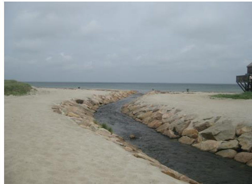
Entrance to creek leading to Bartlett Pond. (BB-02)
