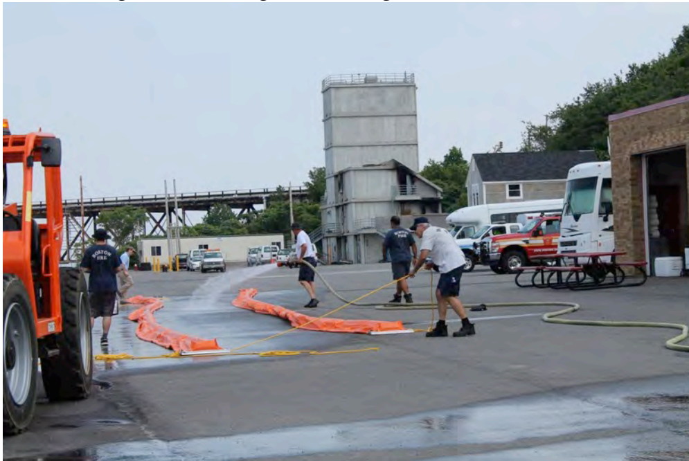
Figure 11. Rinsing Boom during Demobilization Phase
