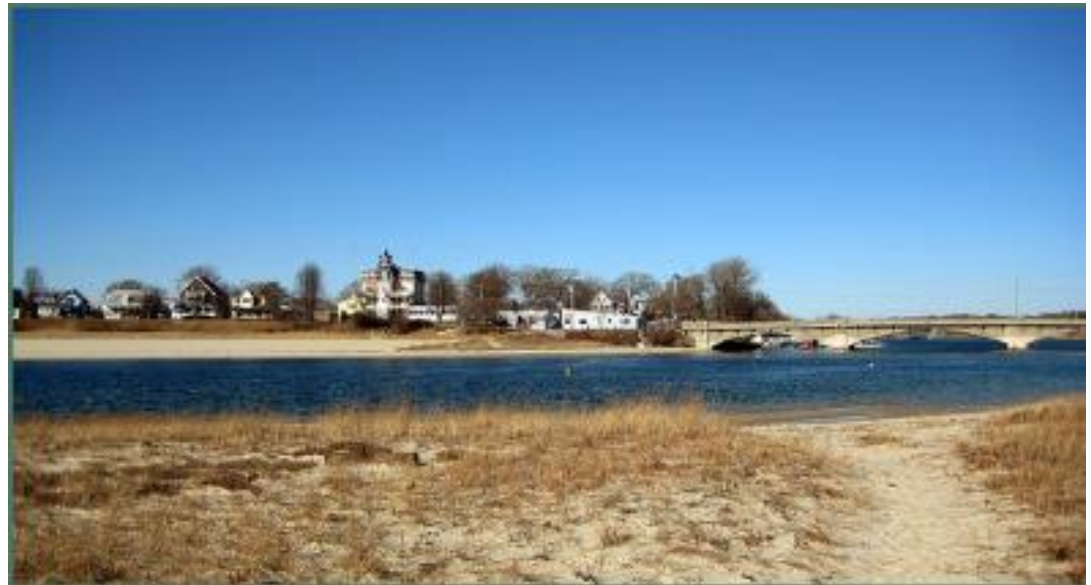
Entrance to East River and Broad Cove (site of DV-01c) looking northwest at mid-tide on 14 Jan 2008.
