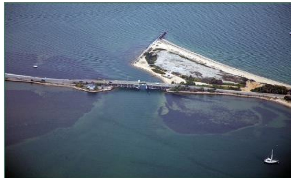
Site of DV-01, Lagoon Pond entrance looking north
