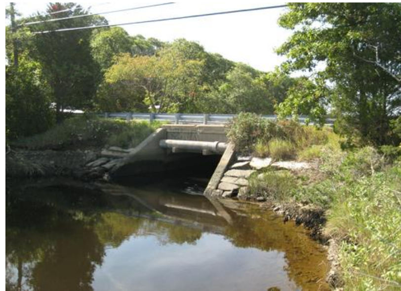
Culvert located along Gannett Rd looking West. Site of CB-01
