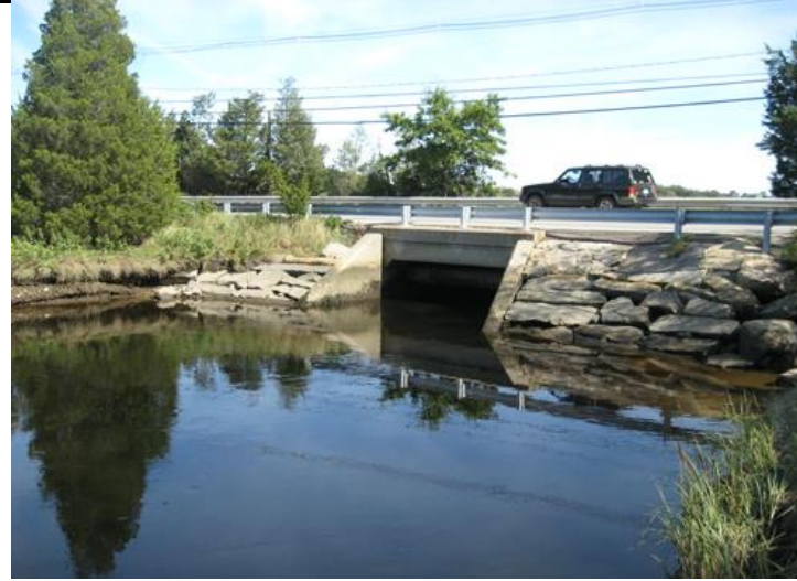
Culvert located along Gannett Rd looking east. Site of CB-01
