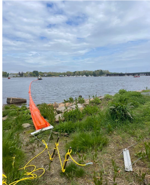
Figure 8: Work vessel drops a marine anchor (background). Shoreside anchor set-up (foreground).
