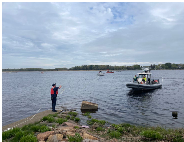
Figure 6: Shoreside crews use heaving line to transfer boom to an awaiting vessel
