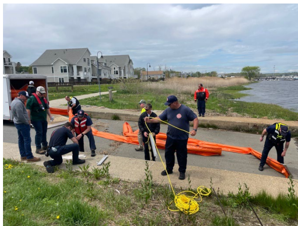
Figure 7: Shoreside crews begin to unload boom from the equipment trailer to configure a shoreside anchor point
