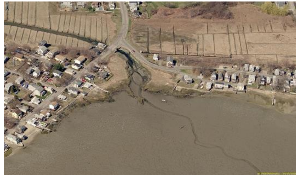
Site of EX-02a, PR-03 entrance to Joseph Street and Spring Street Marshes
