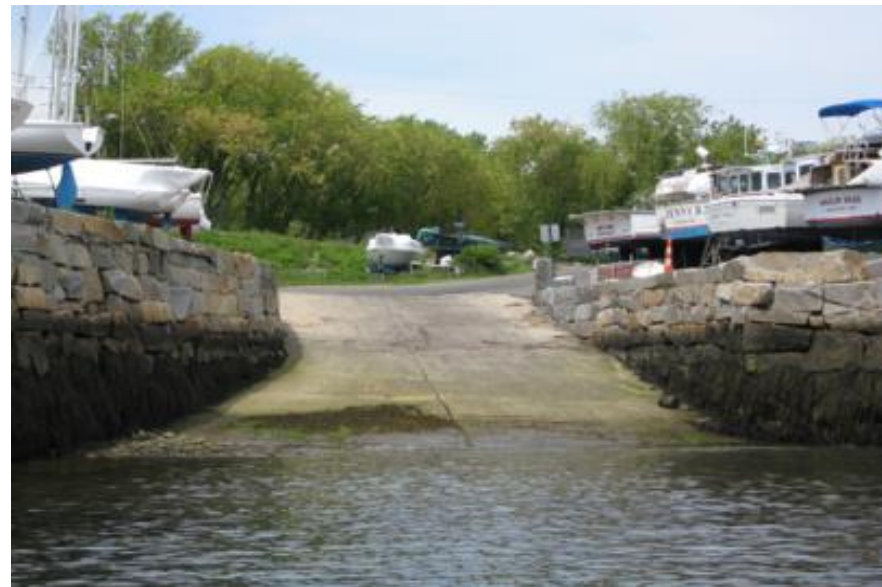
Granite Pier boat ramp at low tide looking north (20 May 2009 photo)
