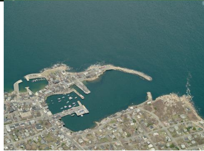
Site of EX-01a, Rockport Harbor (09 April 2009 photo)
