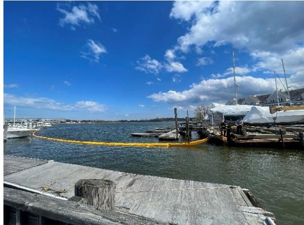
Participants from the shore-side strike team secure end of boom to a pier piling
