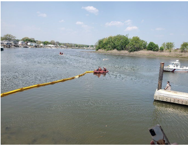
Vessel crews begin towing boom to the deployment site
