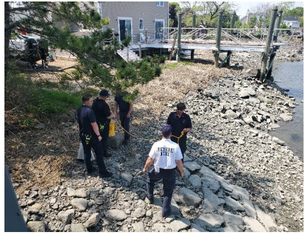
Participants from the shore-side strike team prepare line to attach one end of boom to the shoreside anchor system
