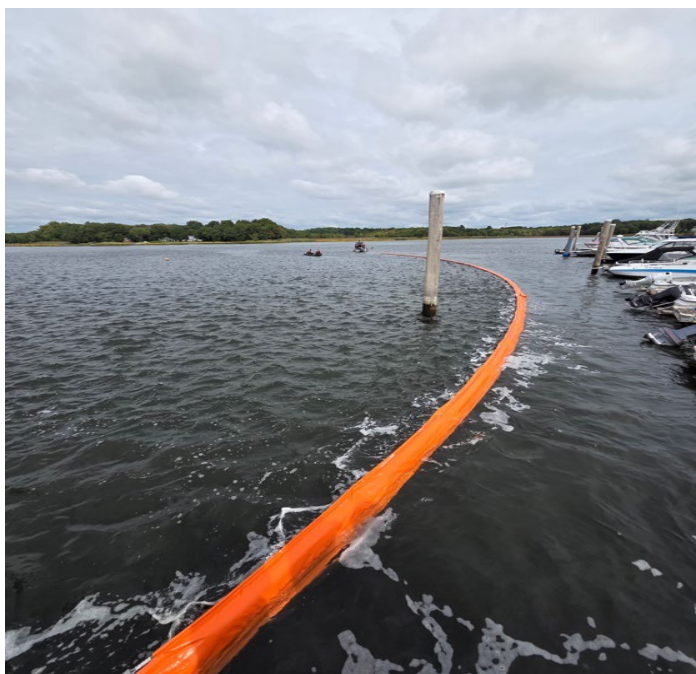
Figure 8: Vessel crews tow the diversion boom against strong currents
