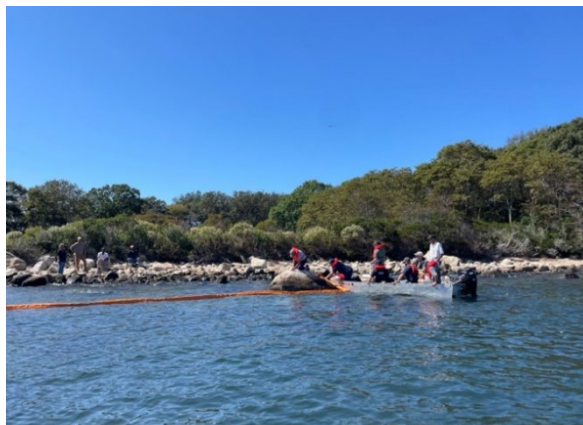
Vessel crews connect boom to a permanent anchor attachment near Bull Island
