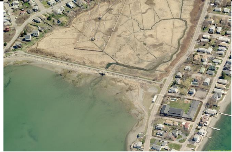
Tide Gate located along Nantasket Road
