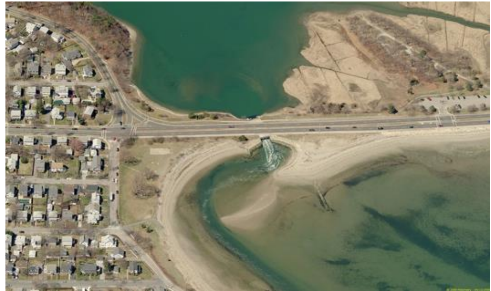
Tide Gate at Blacks Creek
