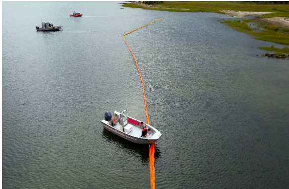
Vessel crews attach an anchor to a section of boom
