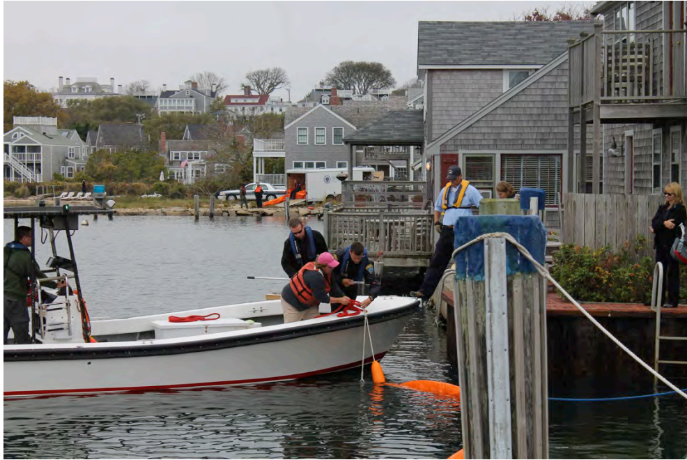
Figure 9. Anchoring a segment of Oil Spill Containment Boom
