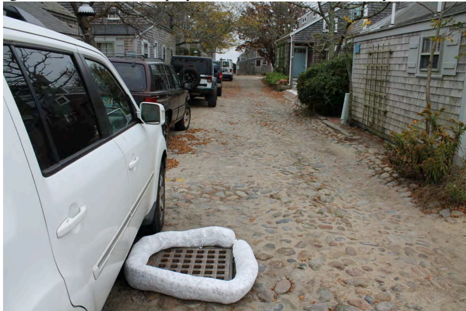
Figure 12. Harbor Fuel deploys sorbent boom around nearby storm drains
