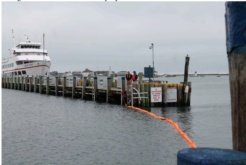
Figure 8. Exclusion boom deployed at Nantucket Boat Basin entrance
