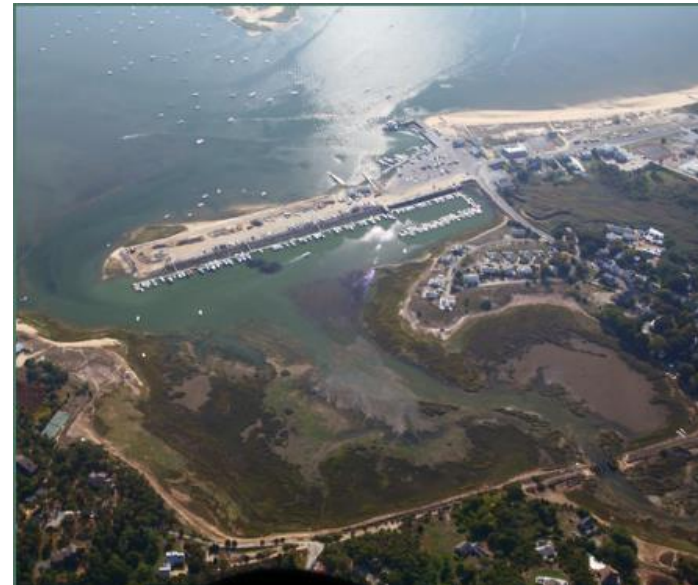
Wellfleet Harbor pier looking southwest
