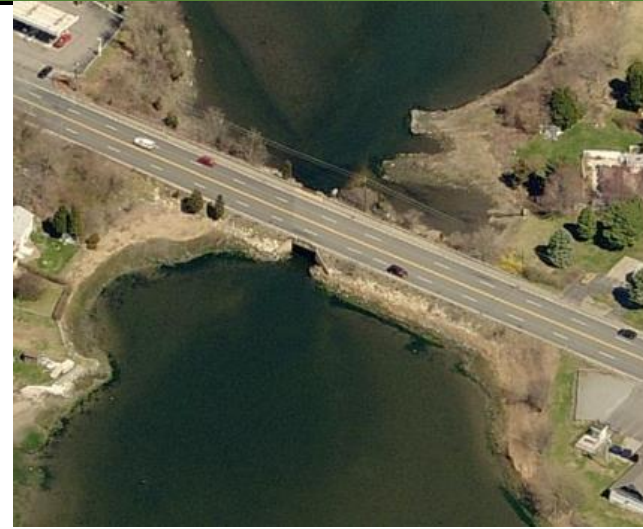
Site of EX-02b at Route 6 Bridge
