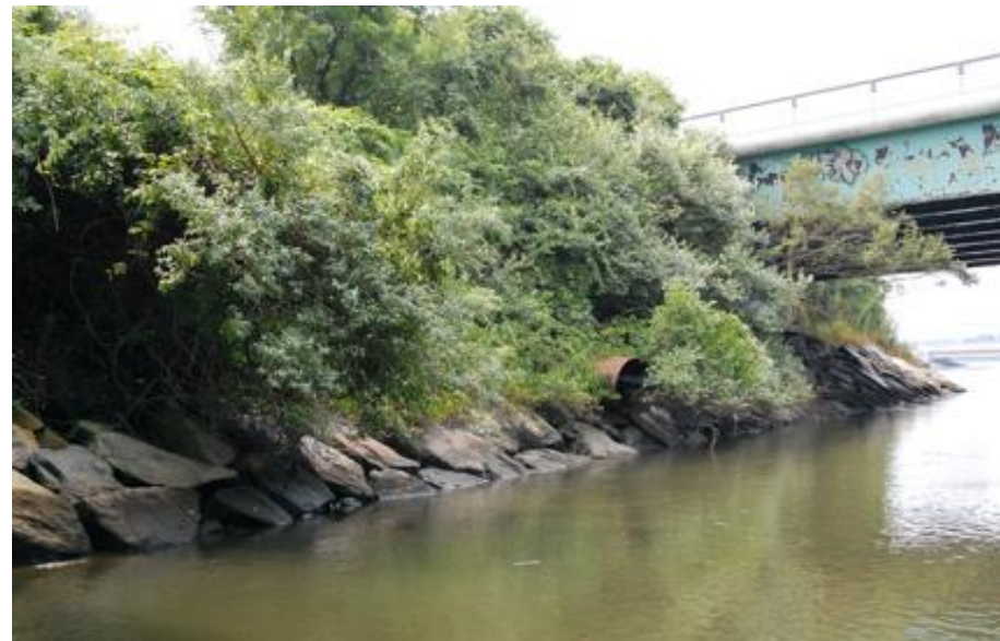
Culvert between I-195 Bridge
