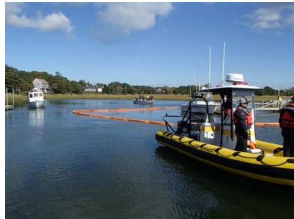
Containment boom around a docked vessel successfully deployed
