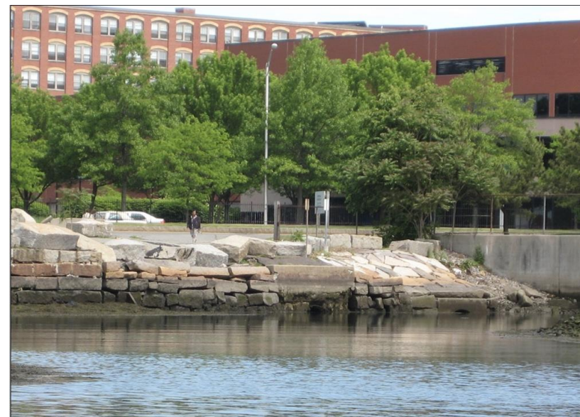
Box culvert at head of Lynn Harbor at mid-tide on 03 June 2009. View looks north.
