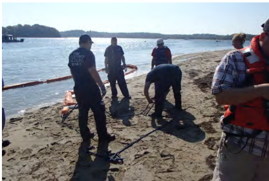
Shore team preparing rebar anchor.
