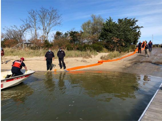
Containment boom around an anchored vessel successfully deployed
