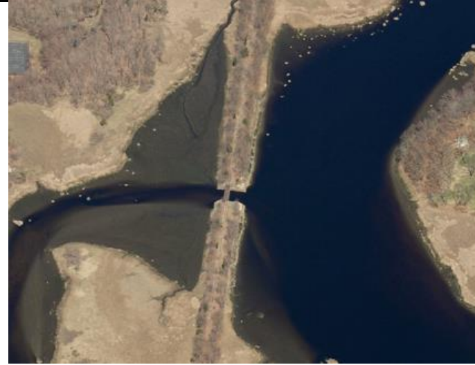
Train Bridge and entrance to Segreganset River (EX-02b)
