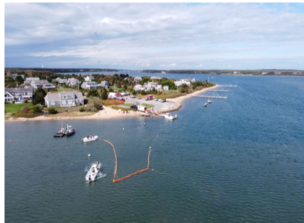
Vessel crew works to deploy containment boom around a mooring
