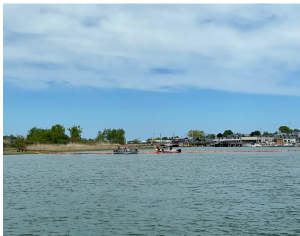
Figure 7: Vessel crew connect two segments of boom to complete the 550 ft diversion array.
