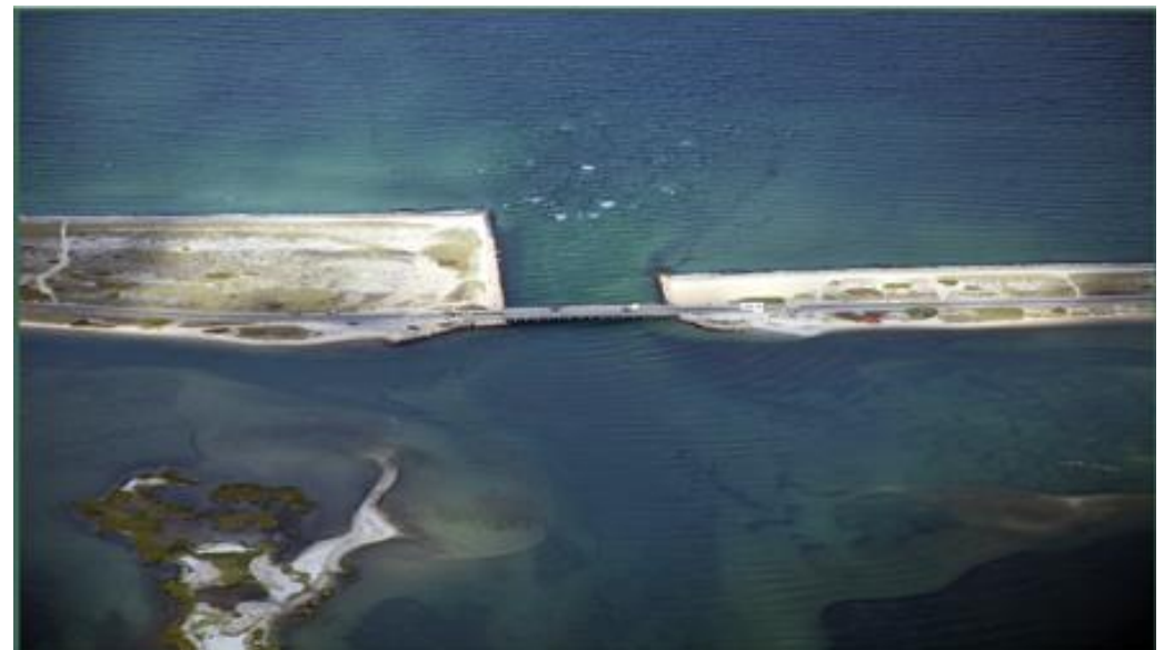
Big Bridge at Sengekontacket Pond looking northeast
