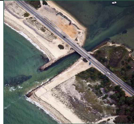
Little Bridge at Sengekontacket Pond looking southwest
