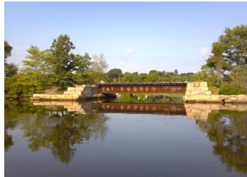
Water level view of Train Bridge
