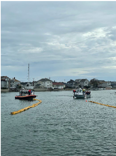
Vessel crews reposition marine anchors on the southern boom section to avoid entanglement in a "No Wake" buoy
