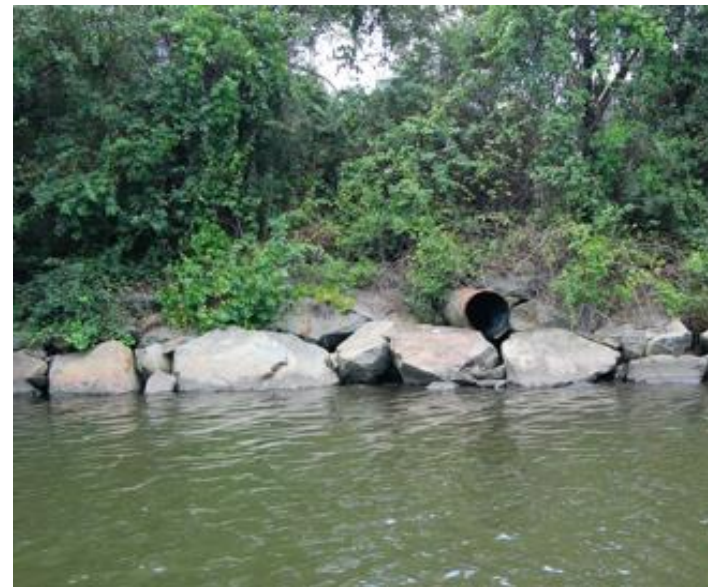
Culvert between I-195 Bridge
