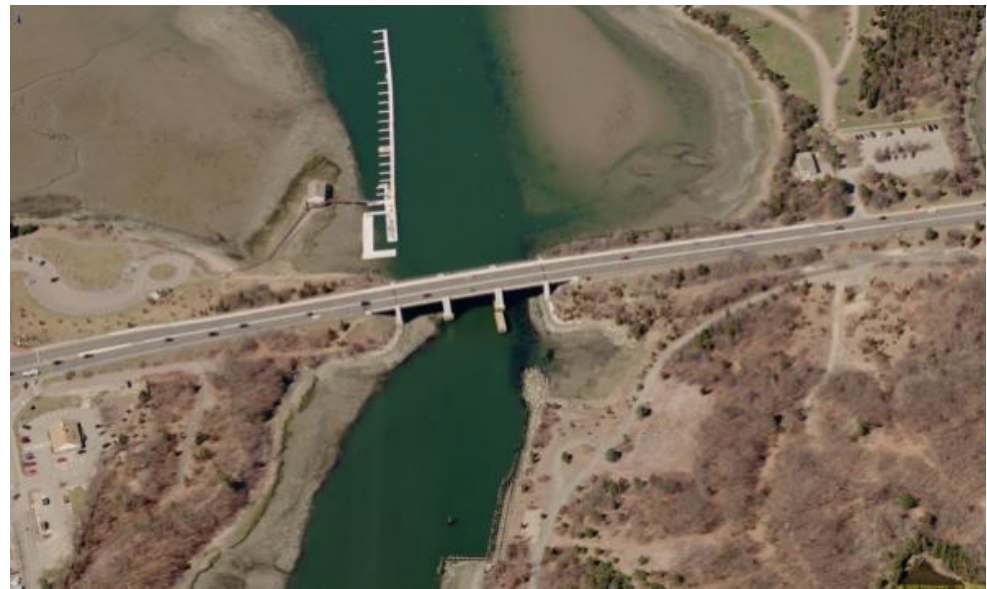
Site of DV-01b looking North to the 3A Bridge
