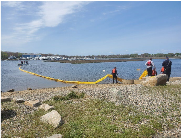
Shoreside anchor crews assist on-water vessels in towing boom to the deployment site
