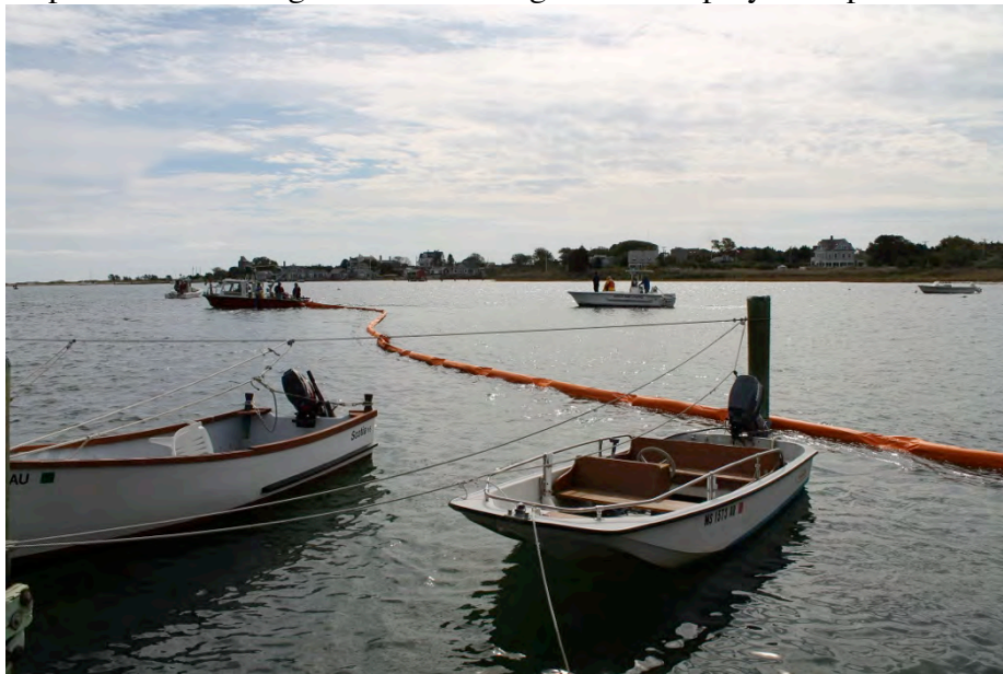
Figure 9. Multiple Towns and Agencies Work Together to Deploy Oil Spill Containment Boom
