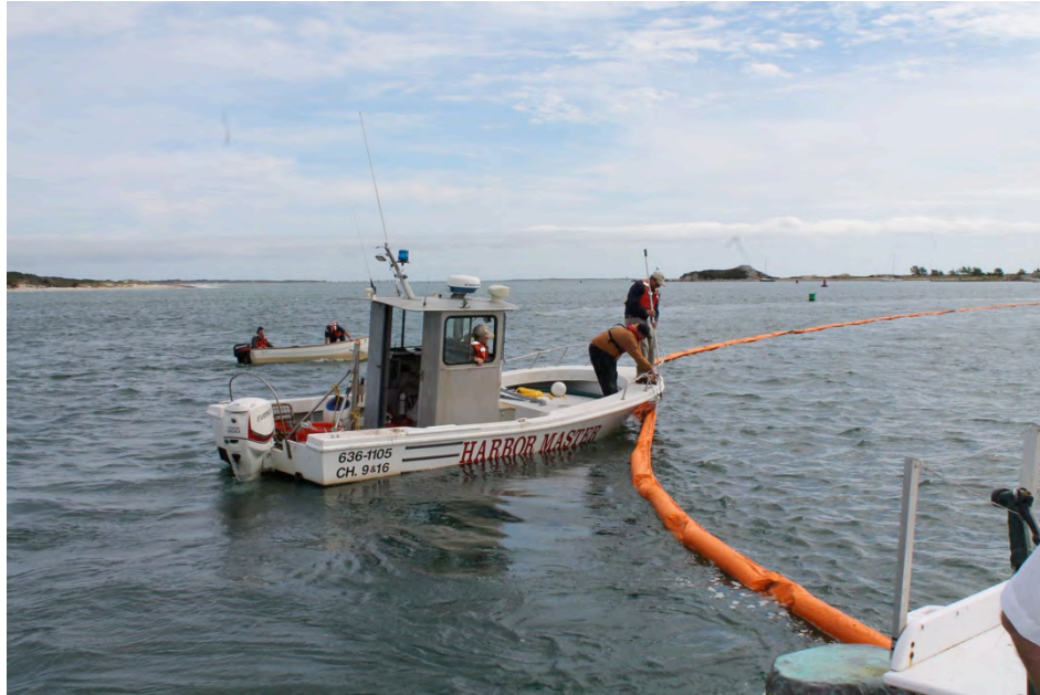
Figure 10. Participants deploy Oil Spill Containment Boom
