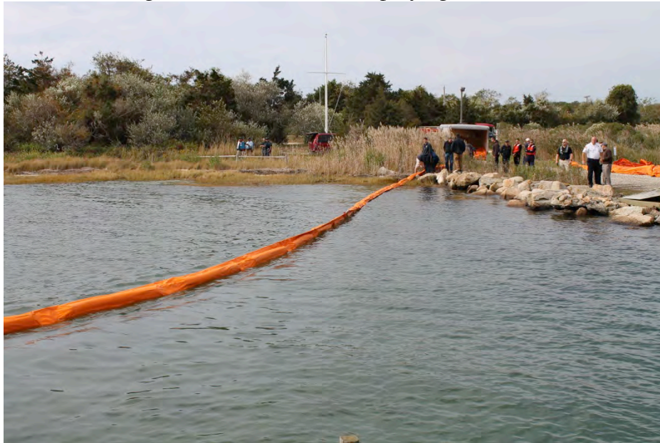
Figure 8. Shoreside crew deploying the boom
