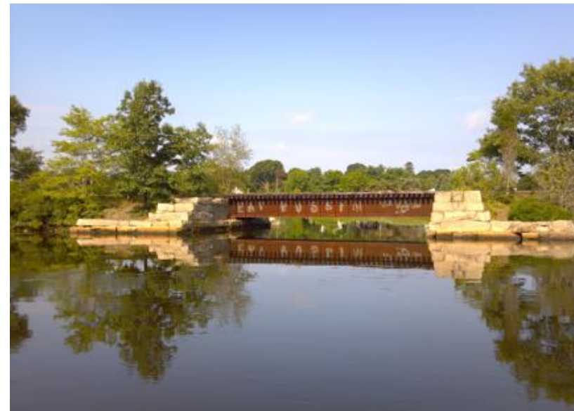
Water level view of Train Bridge
