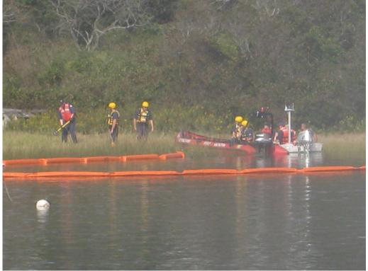
Figure 6. Shoreside Team Anchoring Diversion Boom
