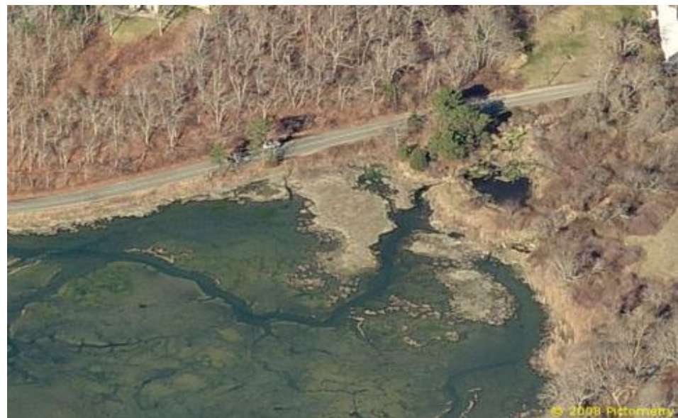
View looking southwest towards culvert near Ellisville Road. (CB-02)
