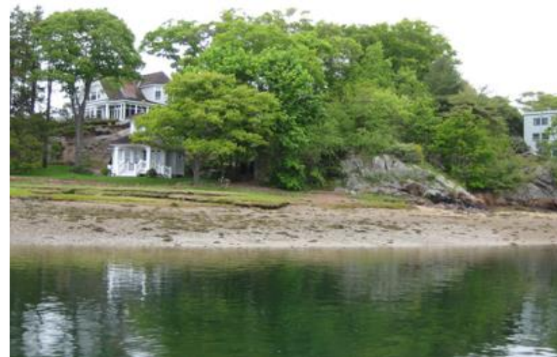
Western anchoring point for EX-02a. View looks northwest
