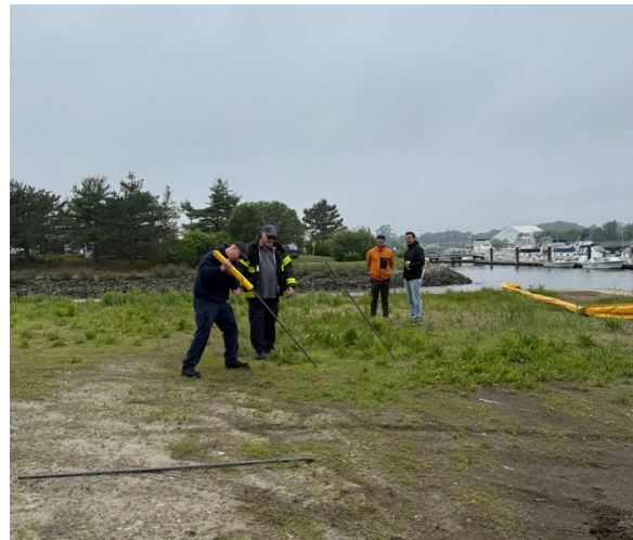
Figure 7: Shoreside crews install a double rebar shoreside anchor
