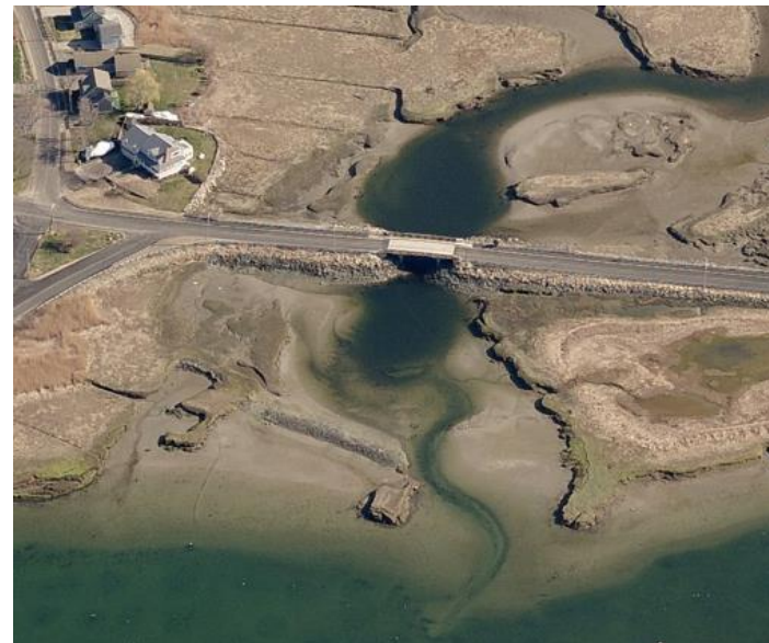
View looking south towards DV-01b
