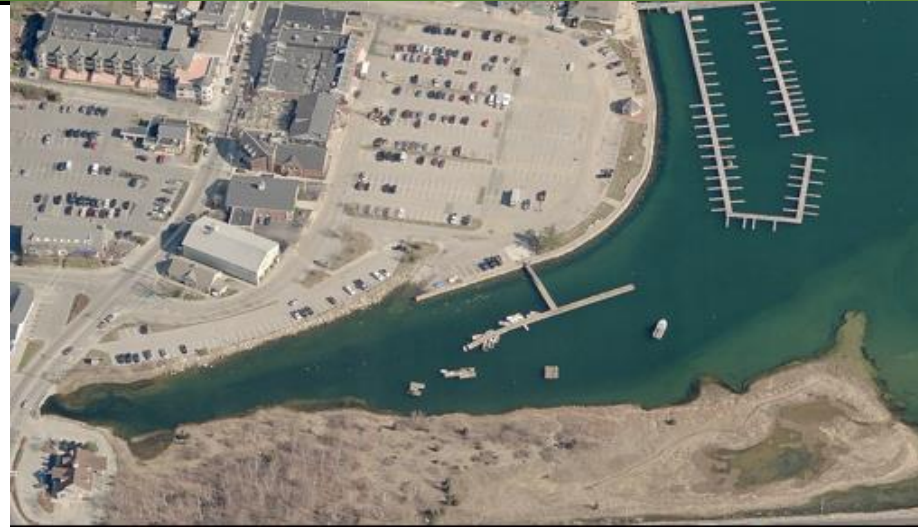
View looking north towards DV-01c
