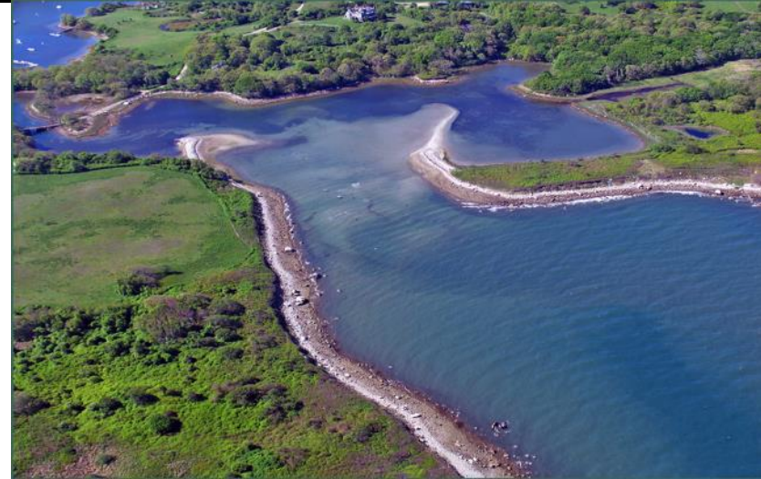
Northwest Gutter looking south at low tide at DV-01a on 29 May 2004. (RPI photo)
