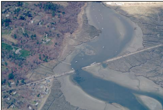
View looking west towards the railroad tracks. (DV-01a & EX-02)
