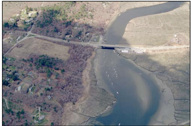
View looking west towards the Rt 3A bridge.
