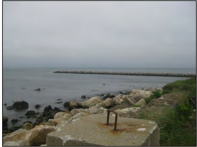
View looking south from the shore of the Pilgrim Nuclear Power Station intake lagoon. (EX-01)
