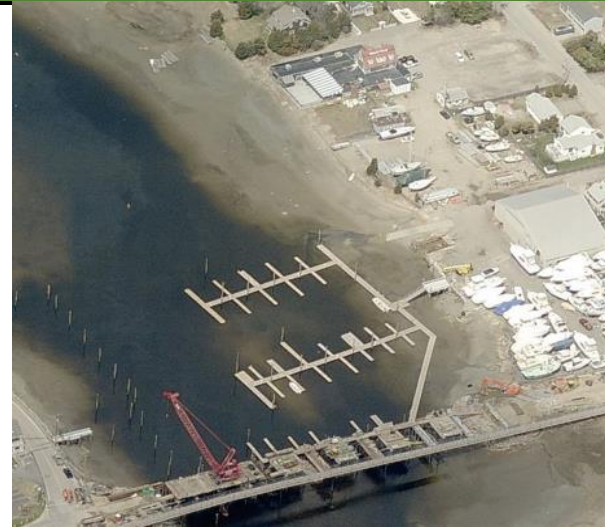
View looking north towards DV-01a and the boat ramp at Humarock Marine Services
