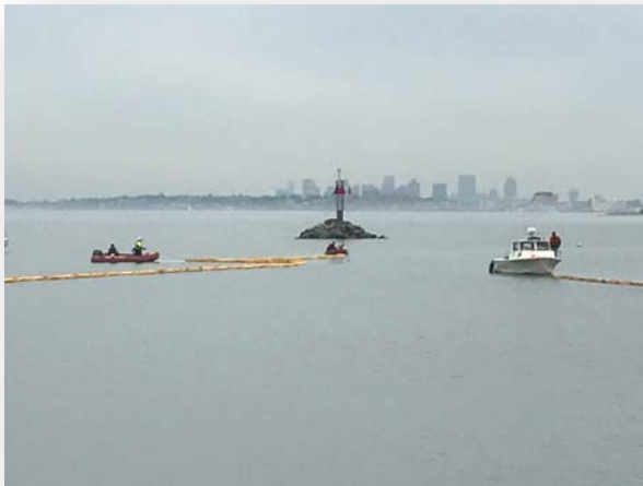
Vessels from Lynn and Nahant deploy oil spill boom in Lynn Harbor.
