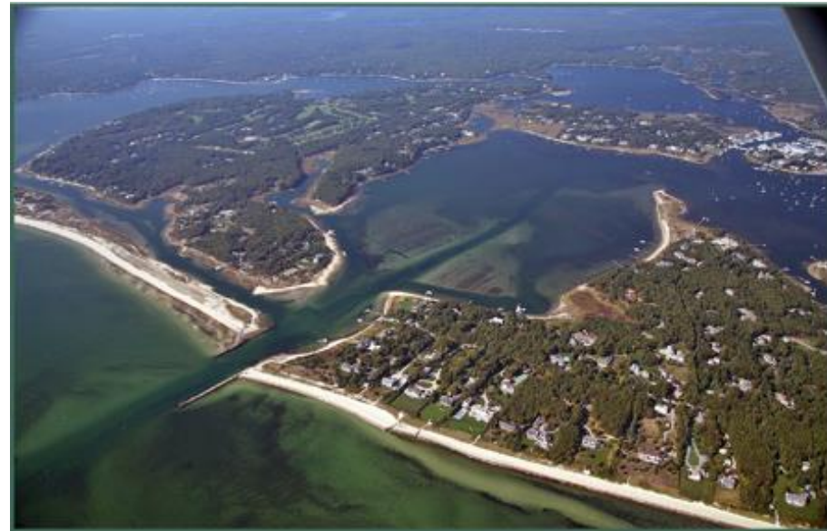
West Bay entrance looking northwest
