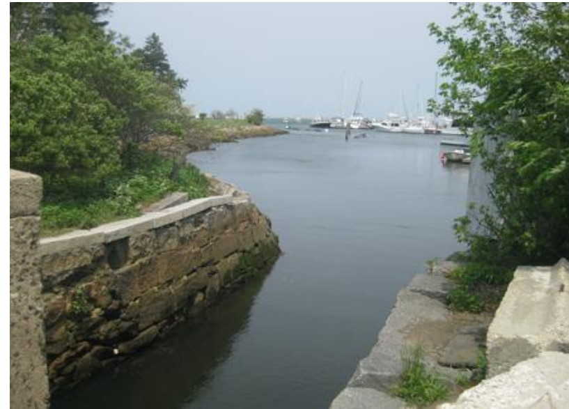
Culvert at Water Street (CB-03)
