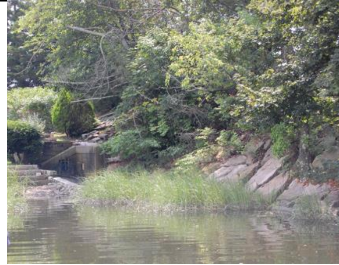
Culvert (note bars covering opening) on Northeast side of MA 103/Wilbur Ave. Bridge
