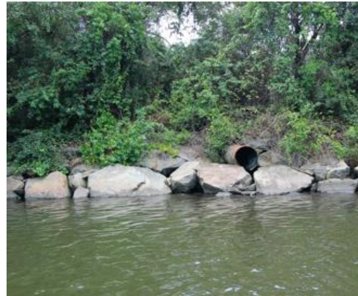
Culvert between I-195 Bridge
