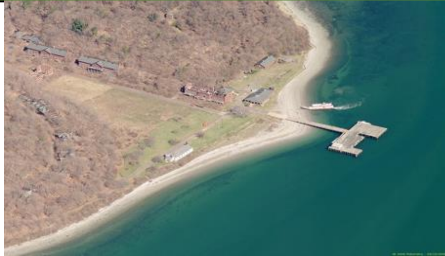
Dock located at the Northeastern point of Peddocks Island
