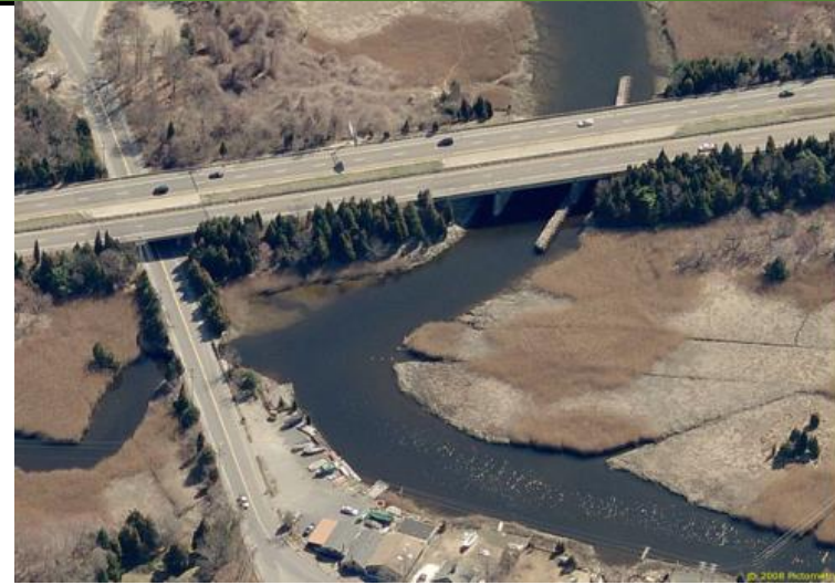
View looking east towards Hwy 3 bridge. (EX-02a)
