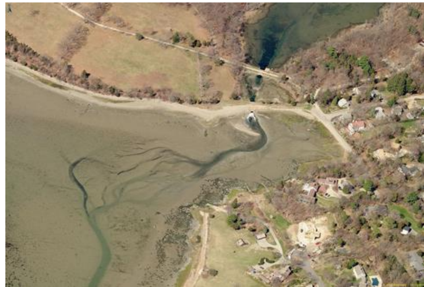
Culvert at CB-02b
