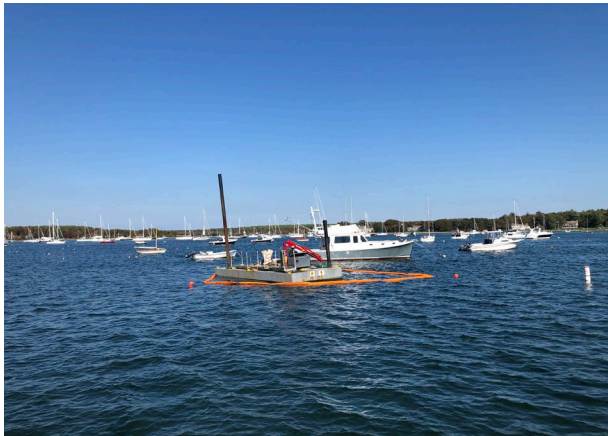
Containment boom around the anchored dredge successfully deployed
